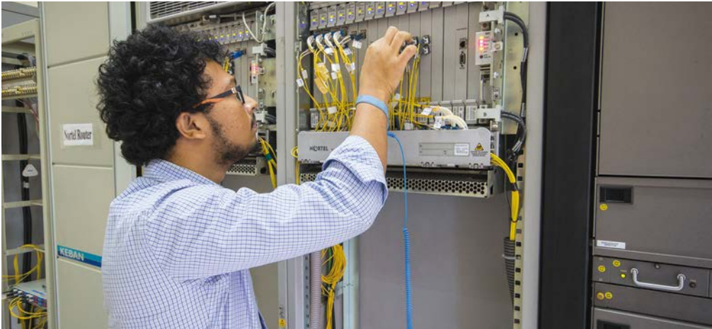
Installation equipment at the cable terminal in Cox's Bazar.
