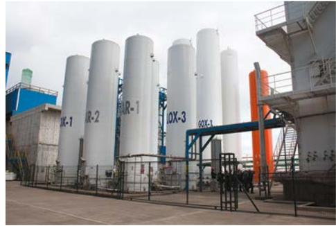
Storage tanks for oxygen, nitrogen gas and liquid argon, part of the oxygen-burning system installed by the Facility.
